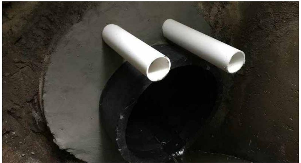
The project was unique in that there was a manhole at each end of the pipe with no way to excavate. NW Relining was able to provide 16-inch, 2.5 foot lengths of Snap-Tite's Thread-Liner that could be lowered into the hole and attached.
